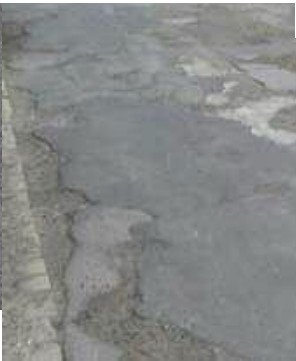
Wearing course deterioration
