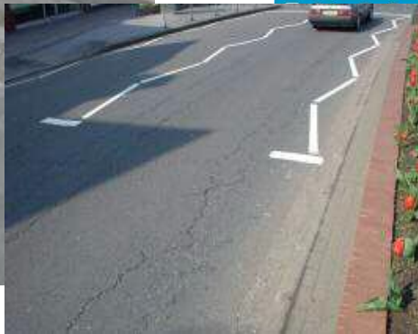
Wheel track cracking
